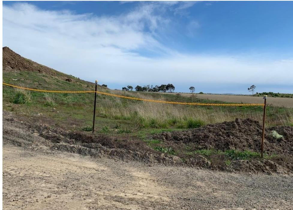
**Figure 2: Yellow chain and star pickets used for delineation of areas**
