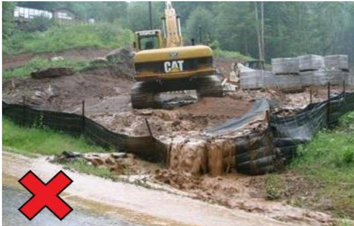
Figure 11: Silt fence failure
