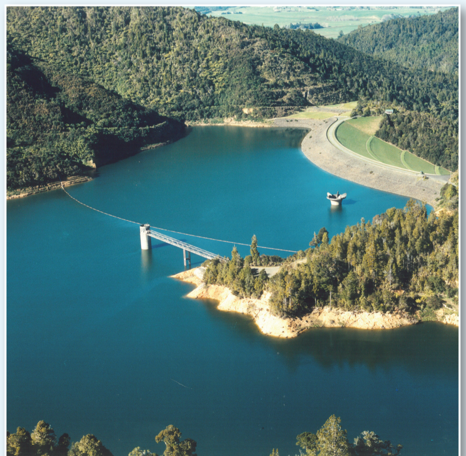
Mangatangi Dam in the Hunua Ranges.
