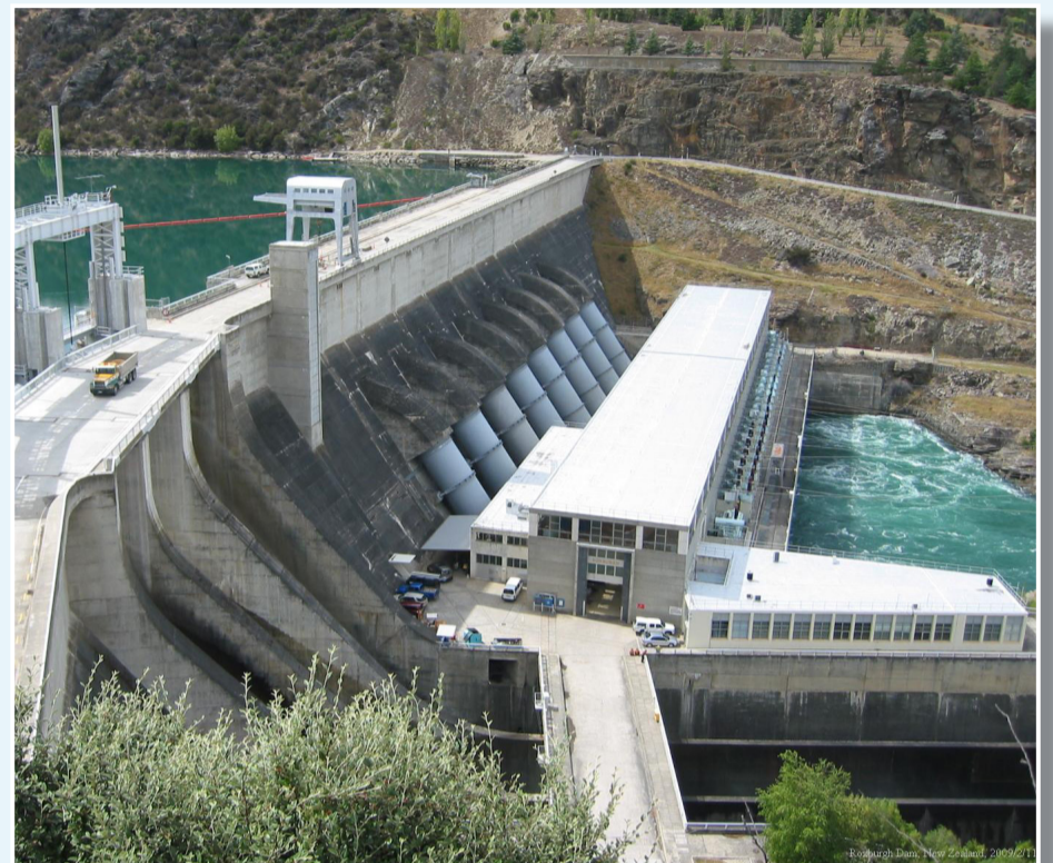
Hydro dam and power station in Roxburgh, Central Otago. Photo credit: Kelisi, Wikimedia Commons.
