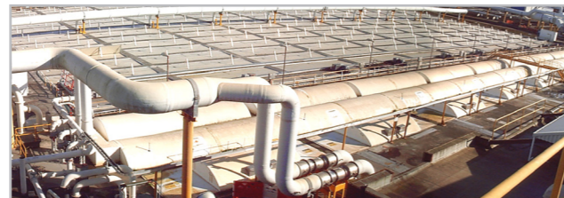
Primary sedimentation tanks
