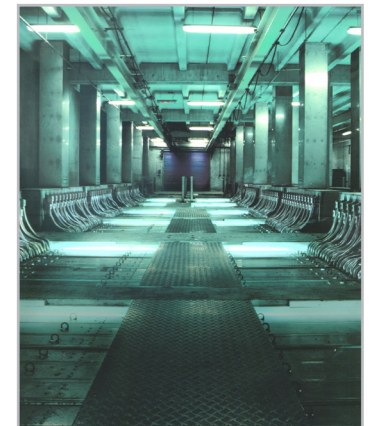
Inside the ultra violet (UV) treatment plant
