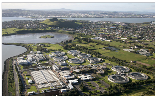
Watercare's Mangere Wastewater Treatment Plant
