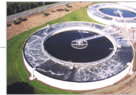
One of the nine reactor clarifiers
