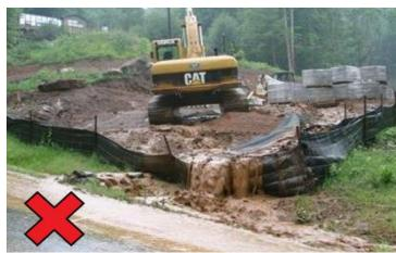
Figure 11: Silt fence failure
