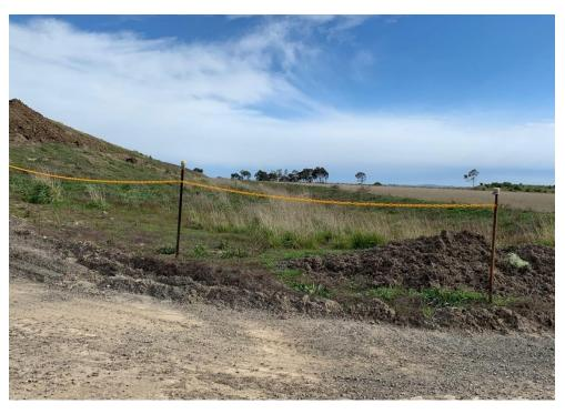
Figure 2: Yellow chain and star pickets used for delineation of areas
