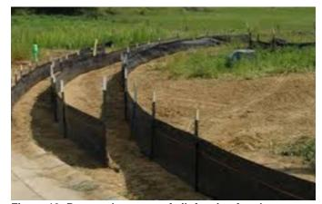
Figure 10: Proper placement of silt fencing for slopes
