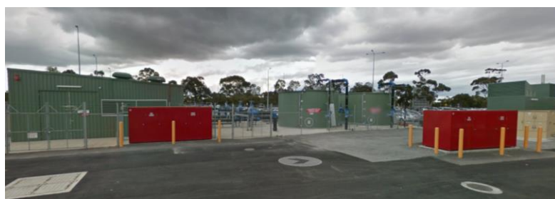
Figure 4.3: Southern Pump Station
