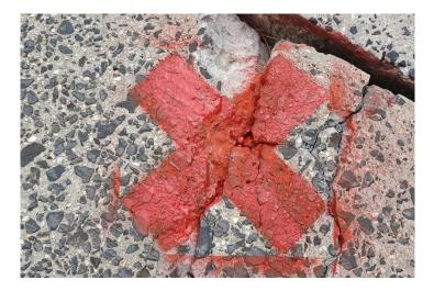
Deterioration of airport facilities contributes significantly to FOD at the airport. Broken lights, spalling concrete and the cork material from concrete joints are all different types of FOD found on the airport.
