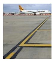
Defines the position where the marshaller is to stop the aircraft nose wheel to ensure the aircraft is parked correctly. It is marked by a solid yellow bar 6 metres long on the port side of the aircraft.
