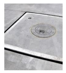
Refuelling Hydrants are marked by a white box. You should avoid driving over the hydrants to prevent both damage to the hydrant lid and damage to your vehicle. Never park on a fuel hydrant.
