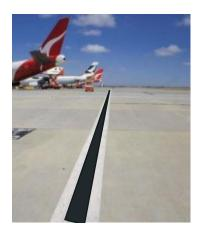
A double solid white line with a black contrasting colour indicating the limit of the ADA Level 2 area, and separating the apron from the Manoeuvring Area (Taxiways and Runways).
