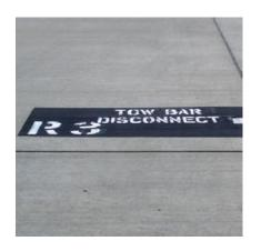
Marked with a white bar – an aircraft is pushed back or pulled forward to this marking. The tug disconnects and the aircraft then departs under its own power.
