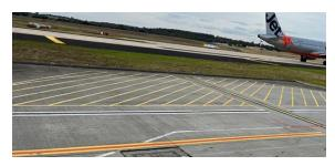
Are indicated by orange hatching. These areas must be kept clear at all times, so the pushback tug has room to manoeuvre when towing aircraft on or off some stand-off positions on the Delta Remote. Level 2 drivers cannot access this area as it is outside the Apron Limit Line.
