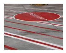
Hazard Areas are marked by diagonal red hatching, usually bordered in white. The marking is used in many areas on the Aprons to signify an area to be kept clear of vehicles and equipment at all times.
