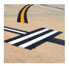
Aircraft are pushed back along the Push Back Line no further than this Limit Line, indicated by two white bars across the Push Back Line.
