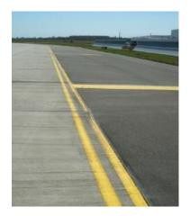
Are made up of double yellow lines on the edge of the taxiway. Extended shoulders are marked with yellow chevrons.
