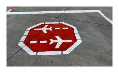
The 'Stop for Taxiing Aircraft' marking is used for taxiway and taxilane crossings between aircraft and vehicles. It means aircraft can cross in front of vehicles, such as on a taxiway or taxilane, entering a parking position under power or when pushing back.
